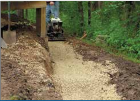
1. Prepare the Site
