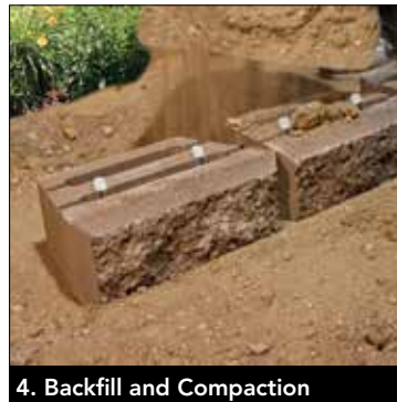
4. Backfill and Compaction
