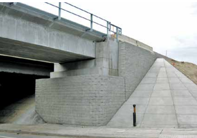
Completed Abutment
