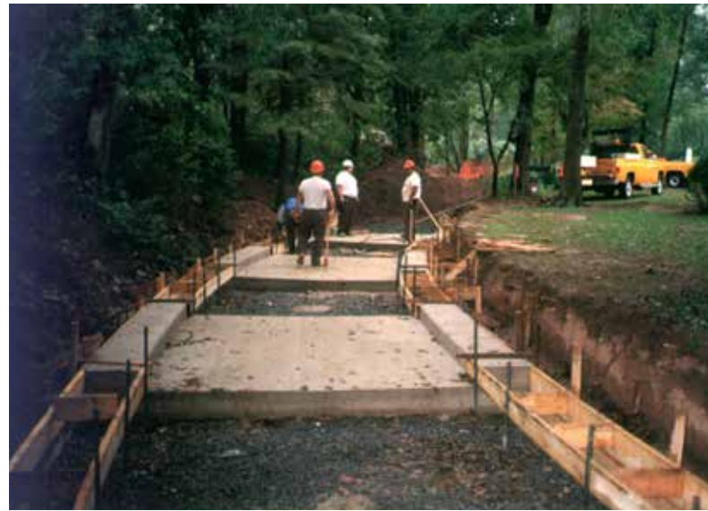
The Keystone units were placed on a concrete footing.
