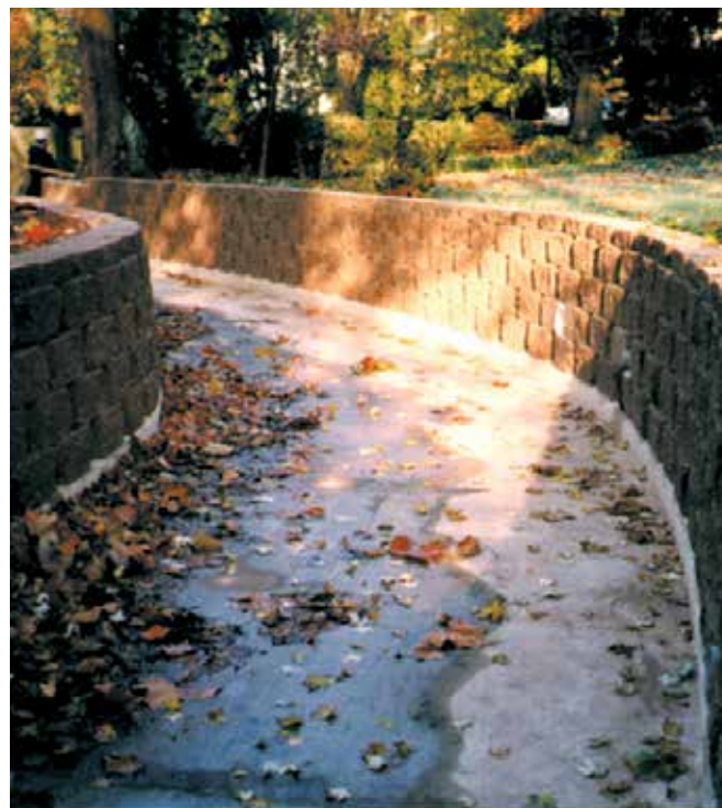
After the drainage ditch improvement project.
