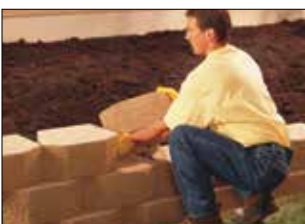
3. Install Additional Courses
