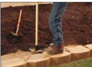
2. Place & Compact Backfill
