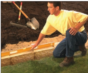
1. Prepare Wall Location
