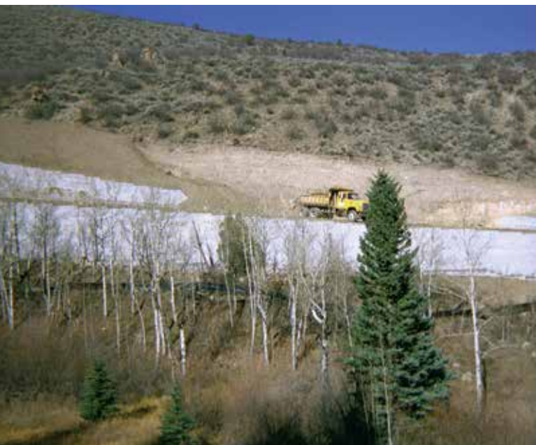
View of completed wall prior to placement of moss stone veneer.
