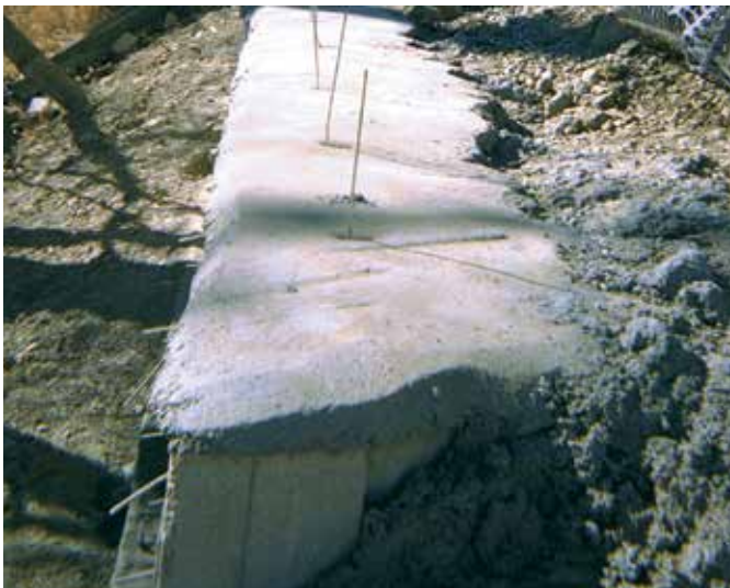
View of top of wall elevation showing grouted cap serving two purposes: (1) seal off water; (2) secure wire to units and provide clean surface for rock attachment.
