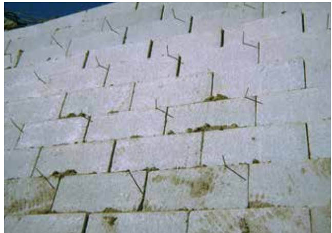
Straight face, unsplit Keystone Standard units with a 9 gauge wire provided the surface and method for attaching the rock veneer.
