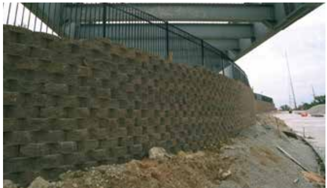
Keystone Compac Tri-plane units were utilized to build this pedestrian walkway.
