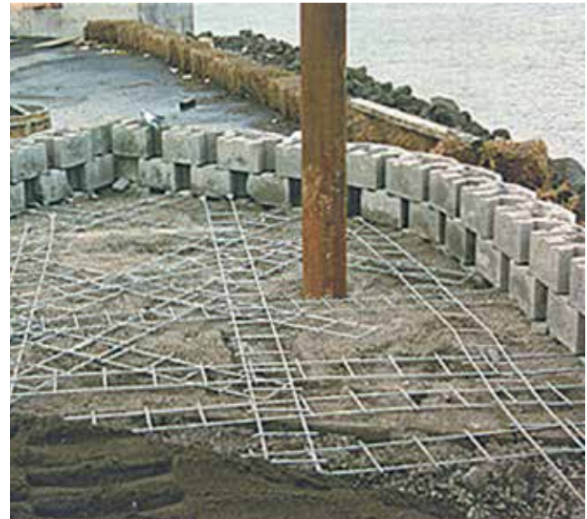
Steel reinforcing layout at bridge support point.
