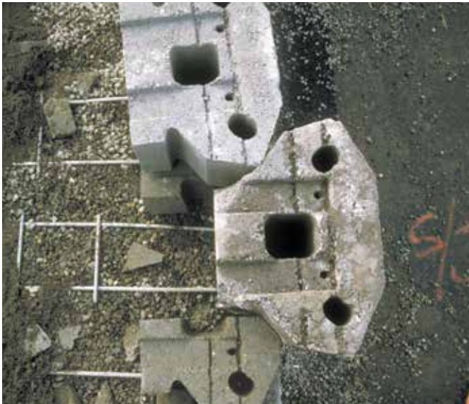
Compac units are cut to fit at vertical slip joints.
