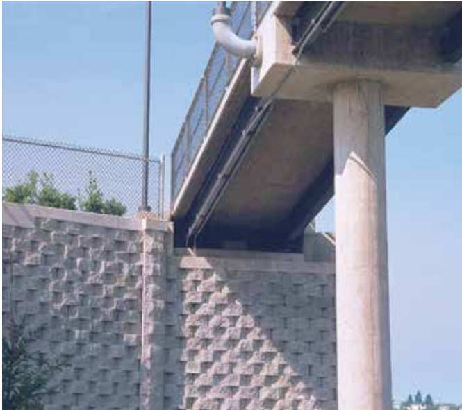
Pedestrian bridge supported by "near vertical" Keystone wall.
