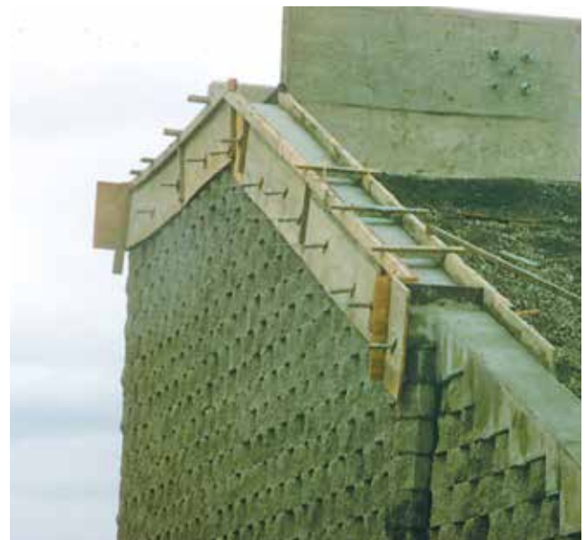
Forming of site poured copings.
