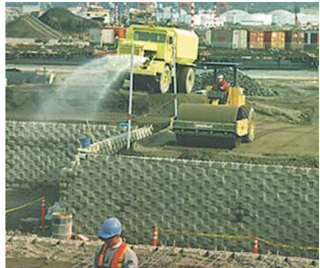
Select granular fill with vibratory compaction.
