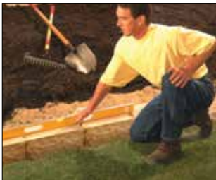
1. Prepare Wall Location
