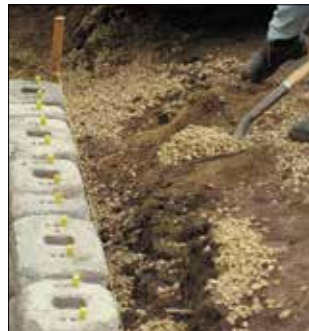
4. Install Fill & Compaction
