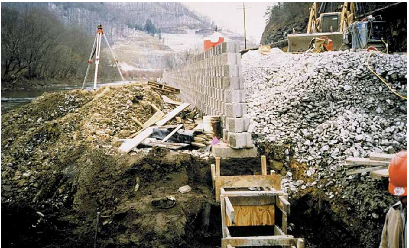
Partial wall shown with forming for additional concrete leveling pad
