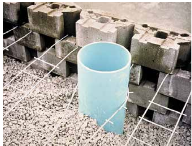
Detail at intersection of vertical post form & KeySteel reinforcement
