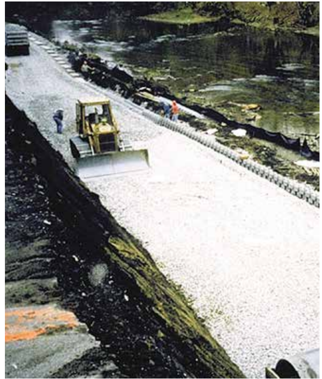
Reinforced fill zone using "select" drainable fill
