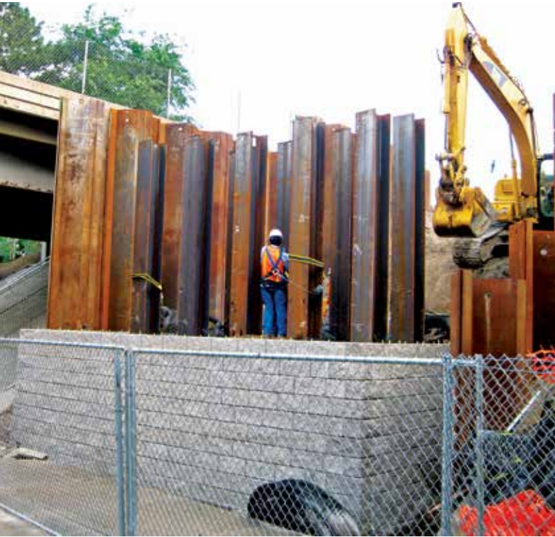
Abutment construction in between interstate bridges
