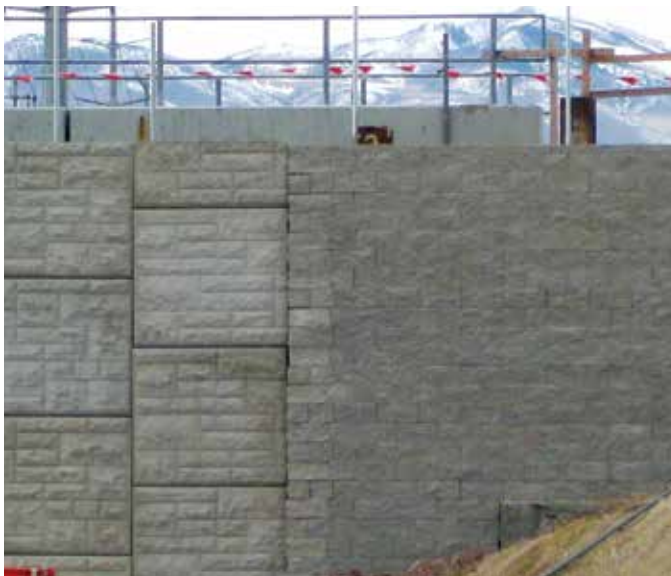
Keystone wall takes over from panel wall system with a smooth transition
