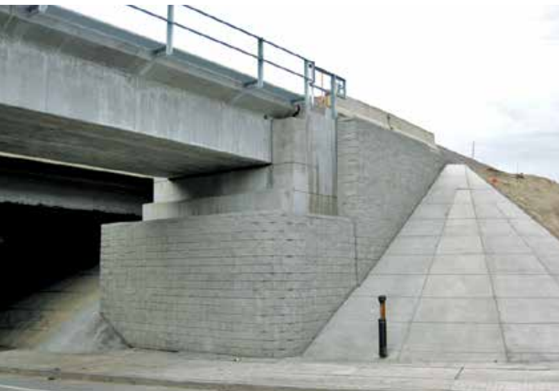
Completed Abutment
