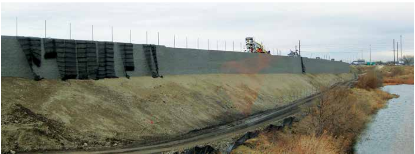
Typical Keystone railroad support walls under construction
