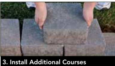
3. Install Additional Courses
