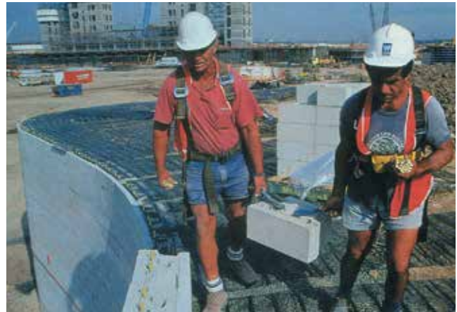
Construction continues with Keystone and geogrid
