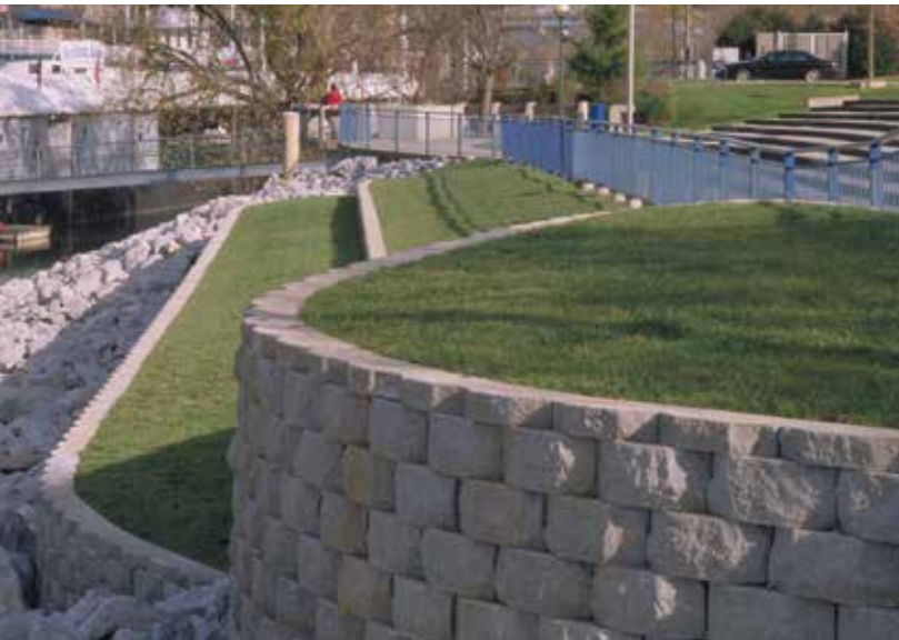
New Terrace wall protects amphitheater from erosion
