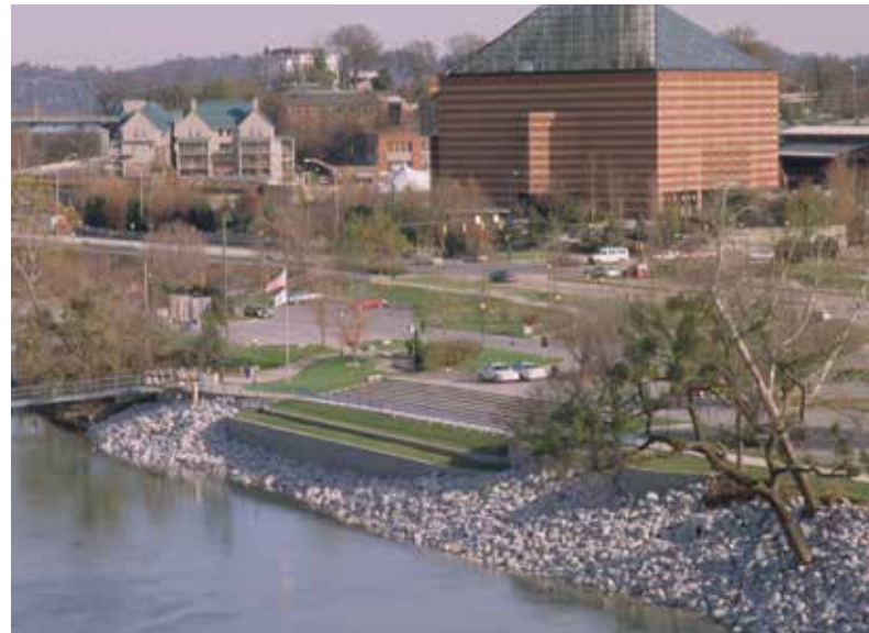
Retaining Wall Solution Protects Park Area
