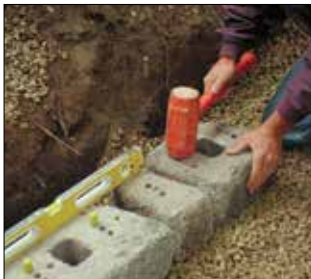
2. Install the Base Course
