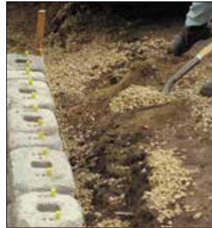
4. Install Fill & Compaction
