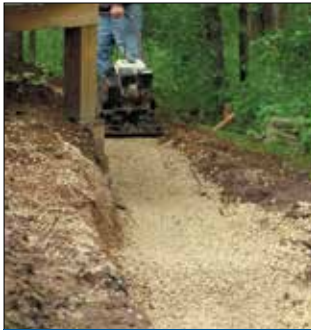
1. Prepare Base Leveling Pad
