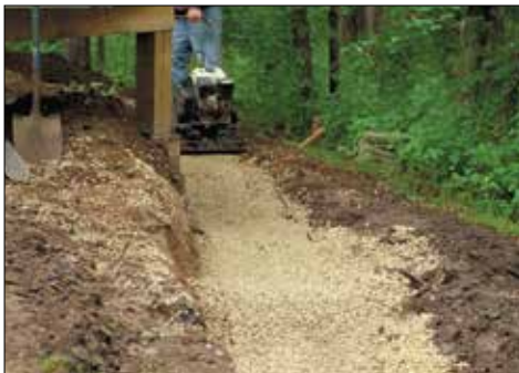
1. Prepare the Site
