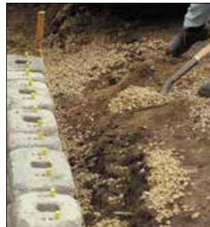
4. Install Fill & Compaction
