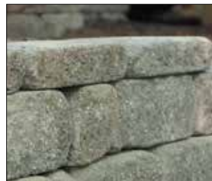
6. Capping the Wall
