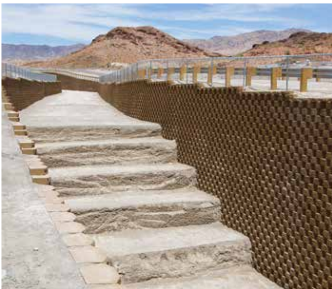
Channel Walls G & F and Access Road
