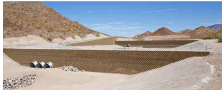
Walls B, C & D and Sedimentation Basins 2 & 3
