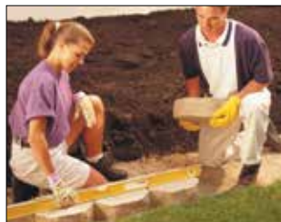
2. Place & Compact Backfill
