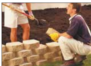
3. Install Additional Courses
