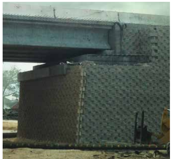
Phased Construction Temporary Wall
