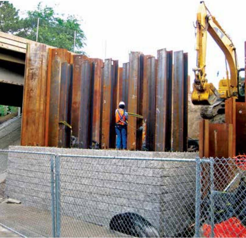
Abutment construction in between interstate bridges
