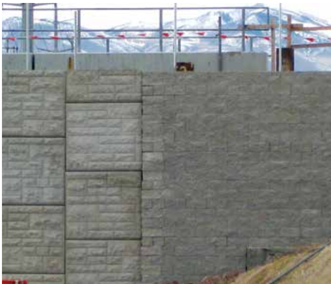
Keystone wall takes over from panel wall system with a smooth transition
