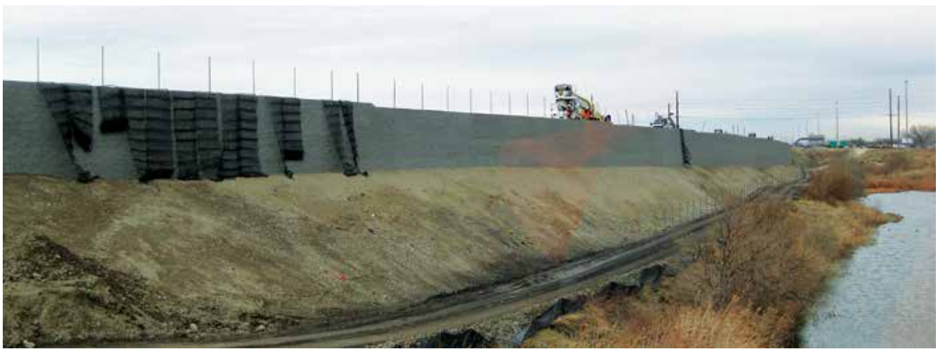
Typical Keystone railroad support walls under construction
