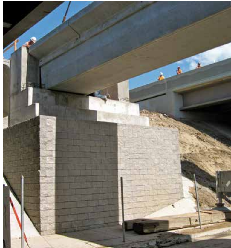
Completed Abutment with beams being set
