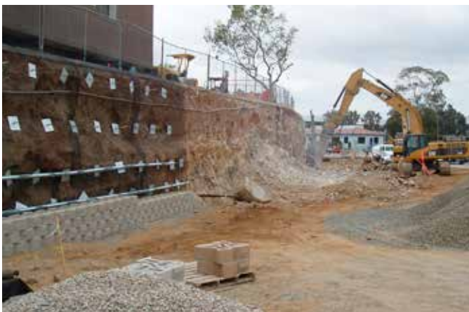
Installing Keystone retaining wall in front of soil nail wall.
