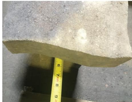
**STEP 2:** Measure the overhang and subtract ½" (equals 5" in this example). This will be the distance that will need to be removed.
