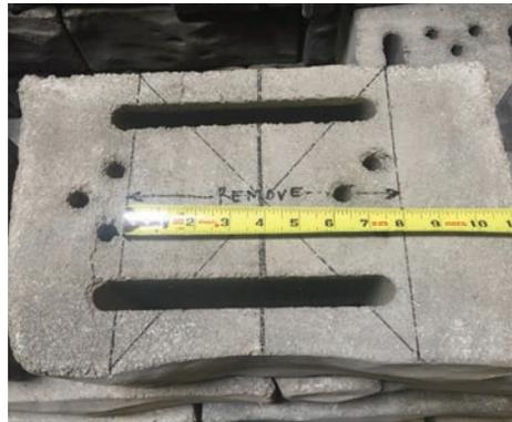
**STEP 2:** Mark a center line on this unit. Next measure half the distance (4") and mark a parallel line on each side of the center line. This will be the 8" that you will need to remove.
