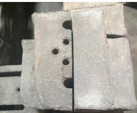
**STEP 4:** Pull the two outside pieces together along the cut side which will be used to fill the 8" opening gap within the wall.
