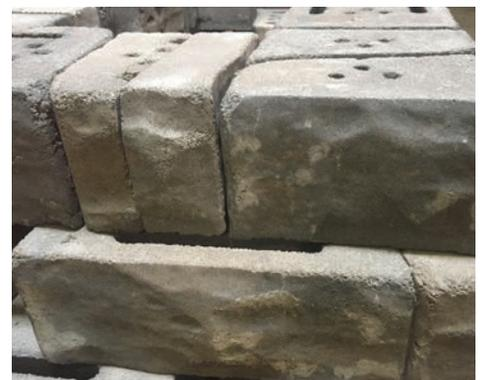
**STEP 6:** Due to the removal of pin holes during the cutting process, these pieces will need to be secured with exterior grade concrete adhesive.
