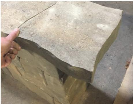
**STEP 1:** Temporarily place capping units on finished wall to determine the amount of overhang.
