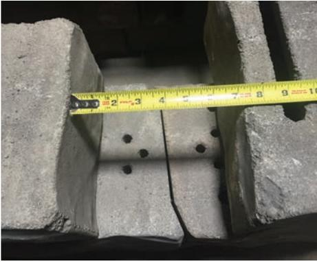
**STEP 1:** Measure the opening gap (7" shown). This will require a 3½" section each of 2 small units.
