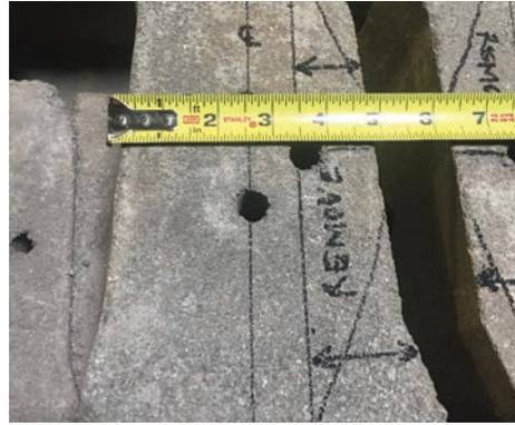
**STEP 2:** On each of the units, locate and mark the center line which will go through the center pin holes. Next, mark a second line at 3½ from textured edge as shown.
