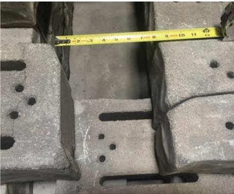
**STEP 1:** Measure the opening gap in your wall (8" shown in this example). Use a large unit (16" wide on long side) to create your cut piece. You will need to remove 8" from the middle of this unit.
