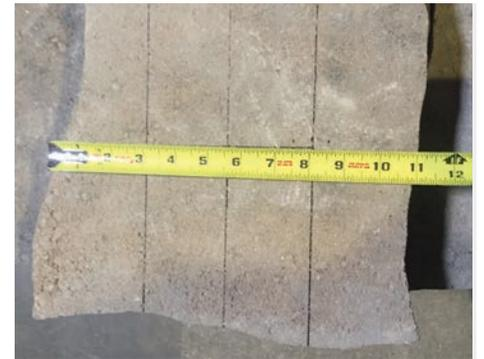
**STEP 3:** Mark a center line on the cap in the direction to be cut. Next, mark two additional lines 2½" on each side of center line. (2½" + 2½" = 5")
