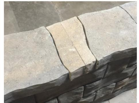
**STEP 6:** For stability and aesthetics, place cut units in the middle of the wall capping and secure in place with exterior grade concrete adhesive.
