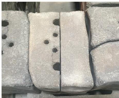
**STEP 5:** For stability and aesthetics, place cut units in the middle of the wall. Line up the cut sides on the textured faces to minimize any offset that may be visible.
