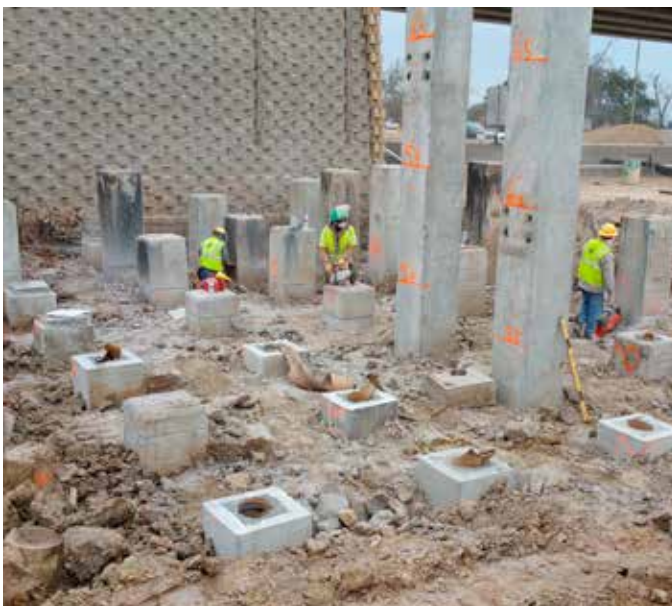
8,000 concrete piles were driven to support the bridge structure.
