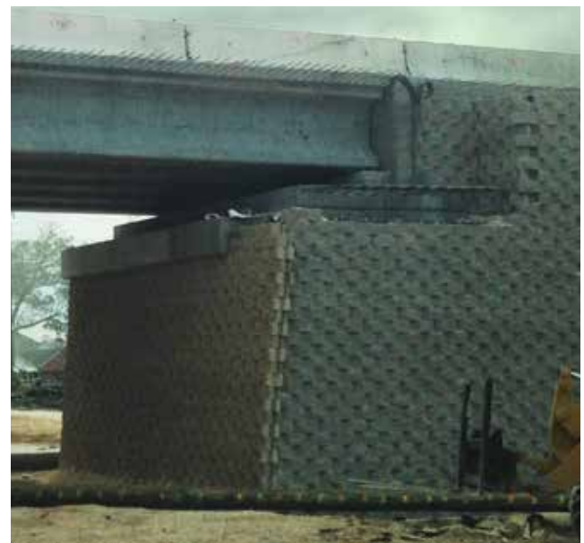
Phased Construction Temporary Wall
