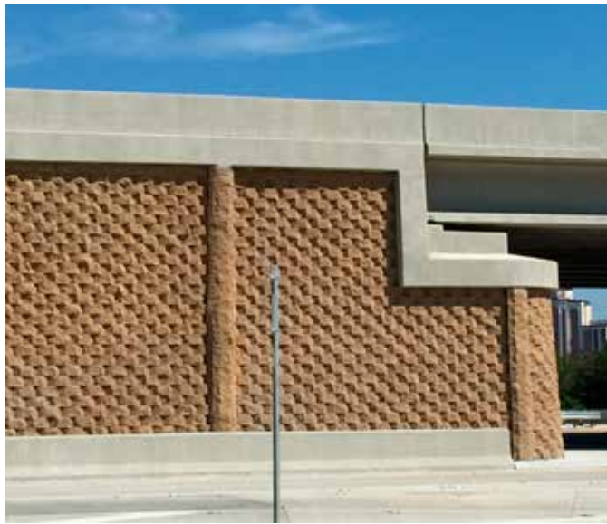
KeyGrid to KeySteel Transition Joint
