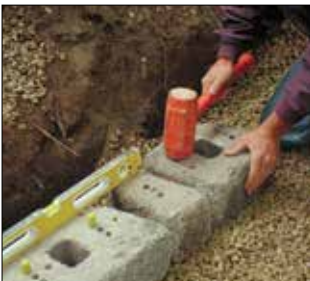
2. Install the Base Course
