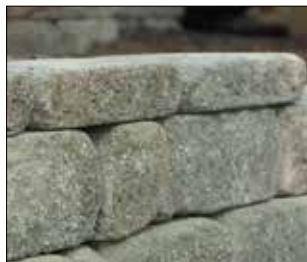
6. Capping the Wall
