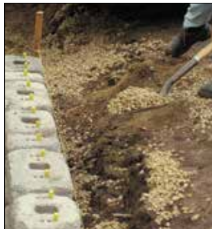
4. Install Fill & Compaction
